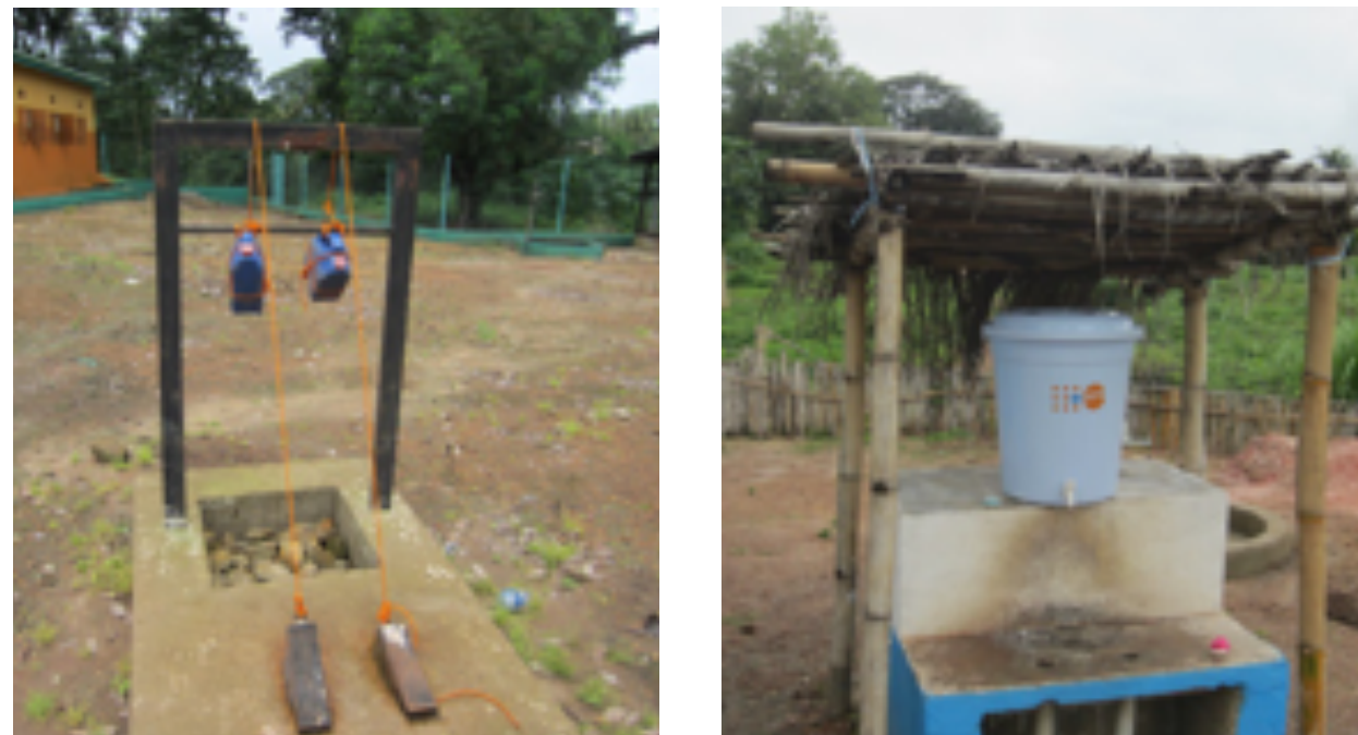
a Hand washing station using pedals (health centre in Guinea)
